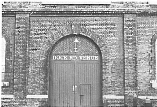
Figure 30: A good example of a sign used to provide a strong focus above the centrally located entrance of a Victorian building.
